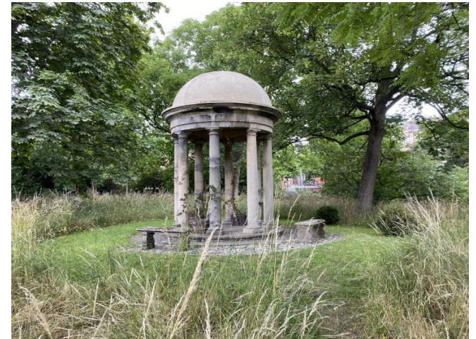
3. Existing structure – structurally sound. Dressed with props and Lambeth benches externally
